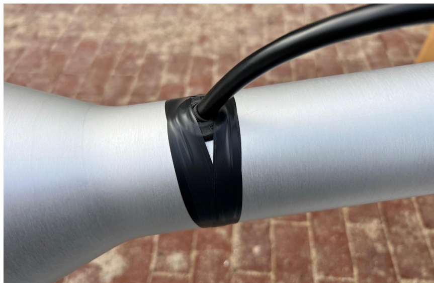
Fig. 7-3: Use Electrical Tape to Secure Cable Grommets
