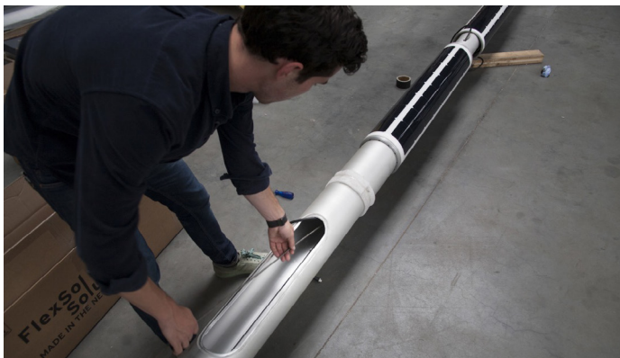
Fig. 9-3: Fish Solar Module Cable to Hand Hole
