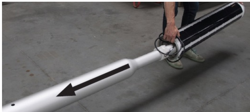
Fig. 8-4: Guide the Solar Module onto the Pole
