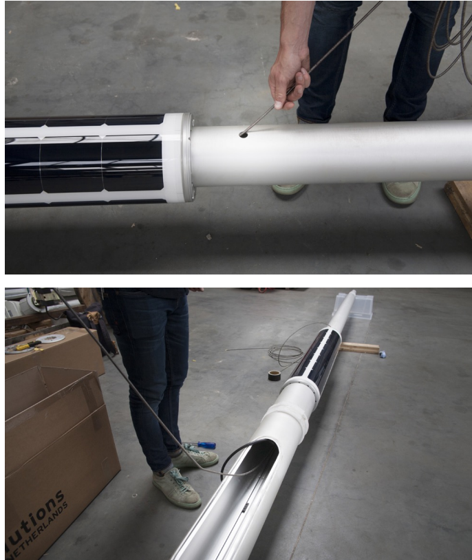
Fig. 9-1: Fish First Solar Module Cable to Hand Hole
