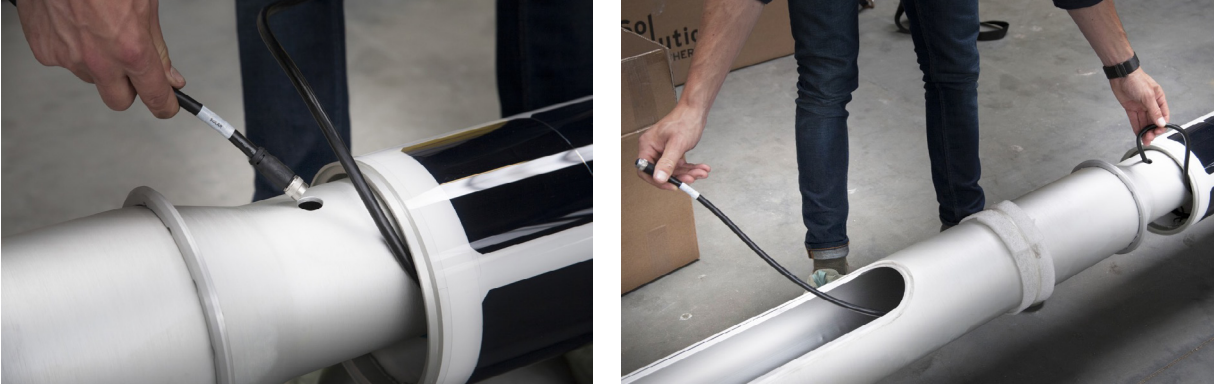
Fig. 8-6: Route Solar Module Cables through Hole on Pole
