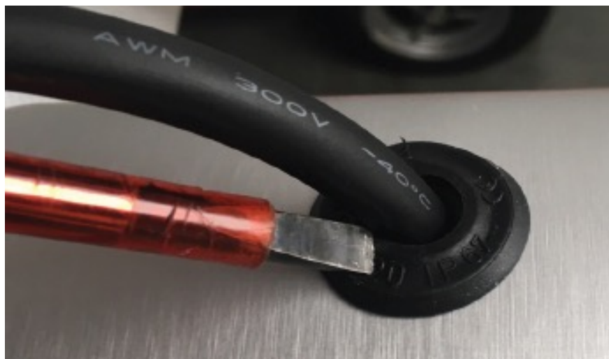
Fig. 7-2: Alignment of Cable Grommet in Hole with Flathead Screwdriver
